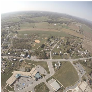
Photo courtesy of Bach's Box.
